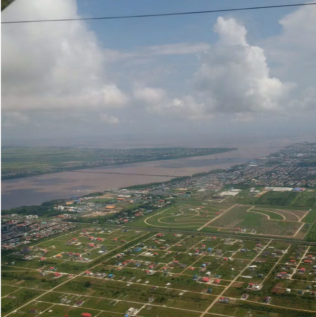
Figure 8.5-5: Demerara Harbour Bridge
