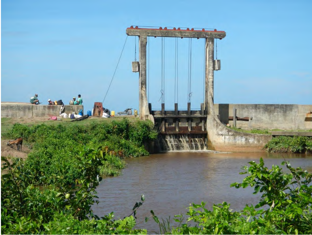
Figure 8.1-8: Sluice Gate (Koker) in Charity (Region 2) at High Tide
